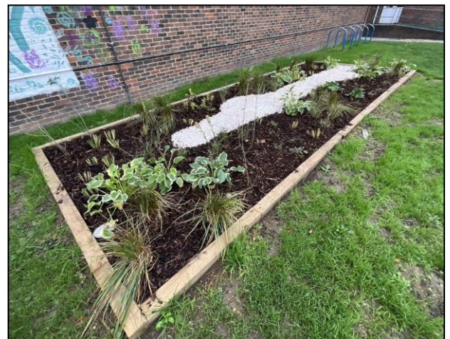
Rain garden constructed
