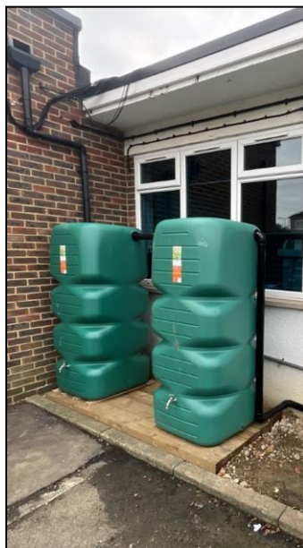
Water butt installation
