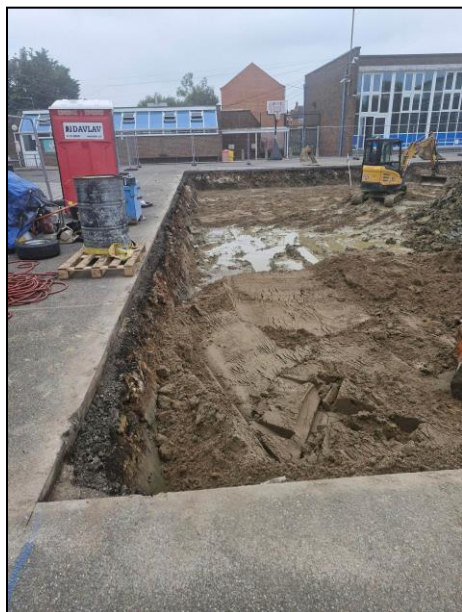
Attenuation tank construction
