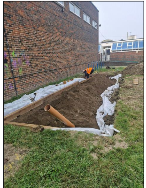
Rain garden construction
