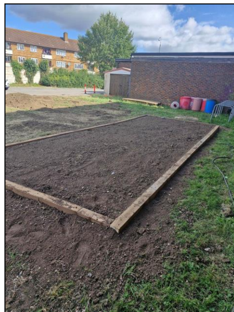
Rain garden construction
