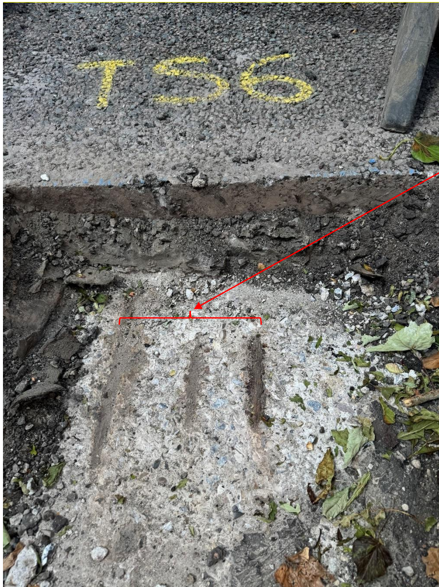
Figure 2- Corroded bars with section loss, possibly due to historic planning, on deck topside -location TS6.
