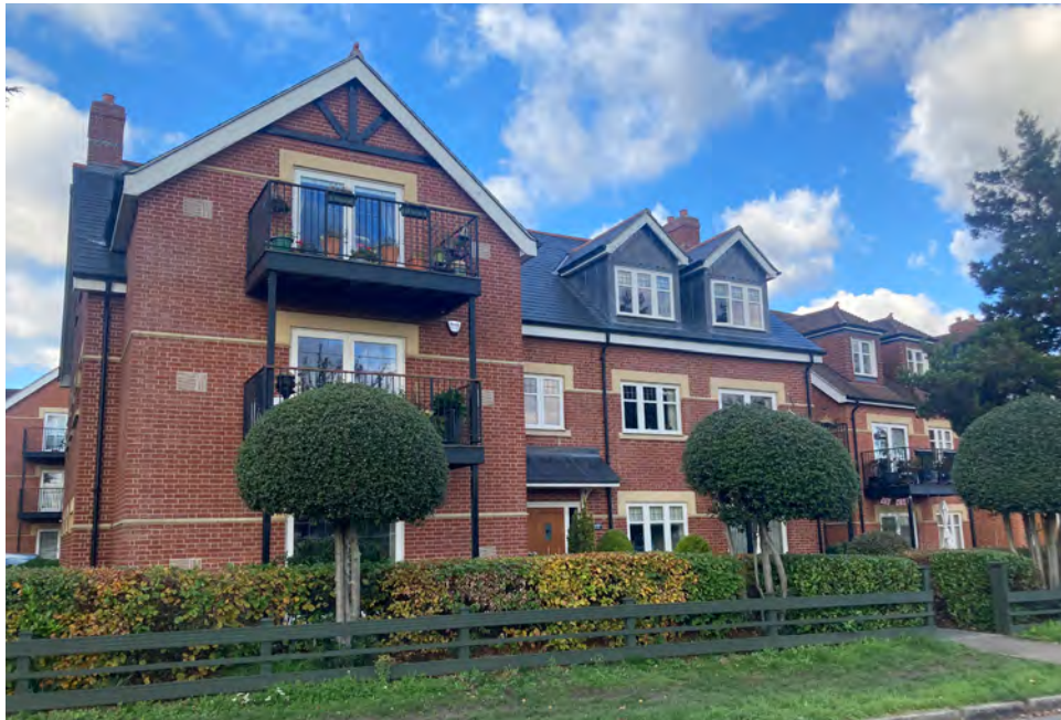
Figure 32 Modern Residential Buildings of north side of Nutter Lane
