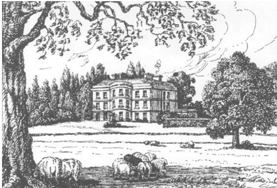
Figure 7 Wanstead Grove House 1690
