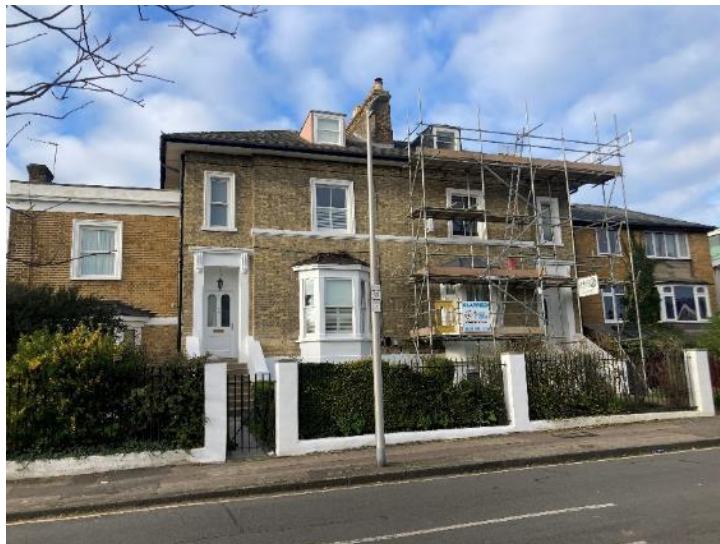
Nos 1 and 2 Grove Crescent
